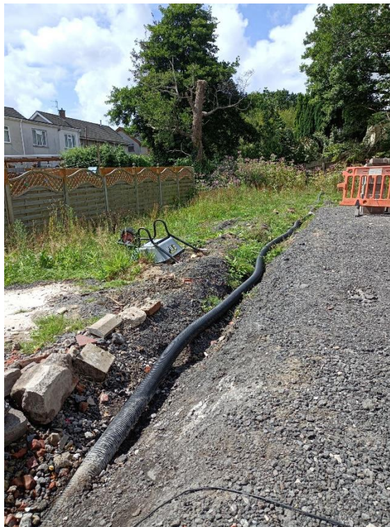
Fig. 5 - Looking towards the rear of the garden –
